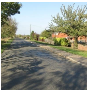
Sutton Road: 40 MPH past houses and Children's Play Equipment
